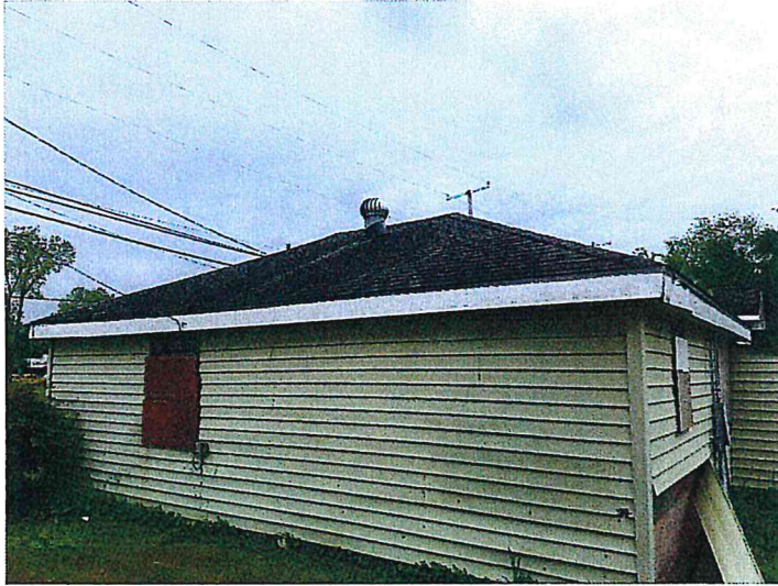
4/19/2016 SAMPLES S57 & S58 - SHINGLE ROOF & FELT MTRL Pic (61).jpg
