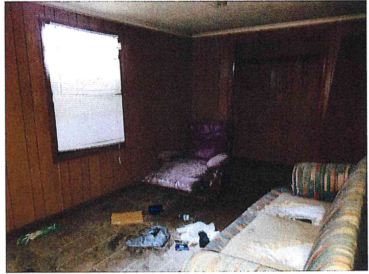
4/19/2016 521 C - INTERIOR Pic (56).jpg
