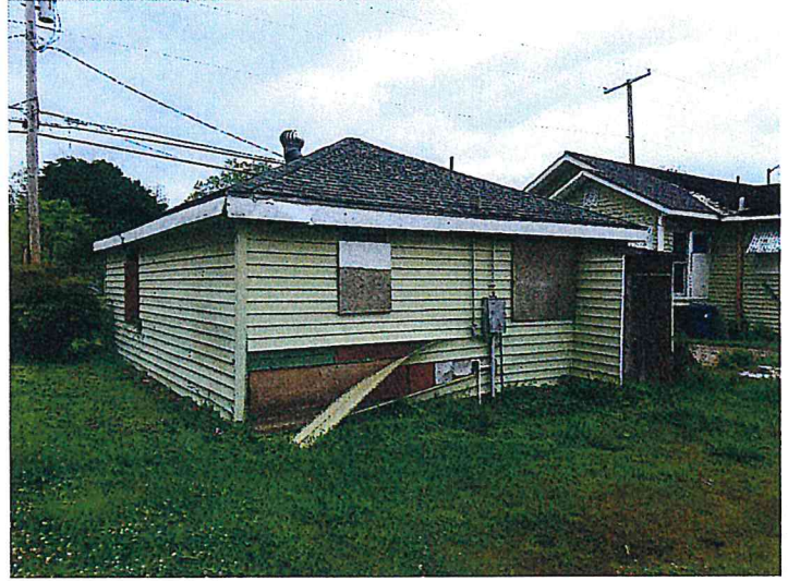
4/19/2016 EXTERIOR SIDES B&C - 521 C NE EVANGELINE THRUWAY Pic (54).jpg
